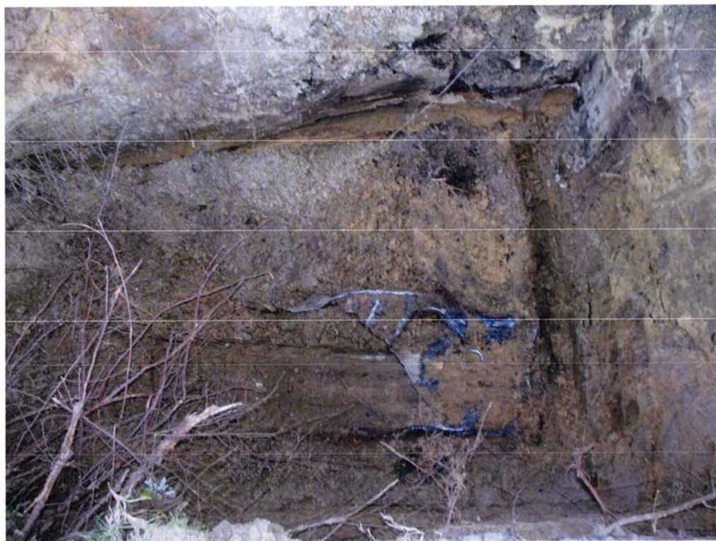
Picture 2: UST 891Cobia excavation in progress.
